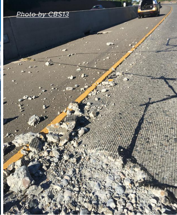
Figure 5: US 50 Pavement Buckling During 2017 Heat Wave
