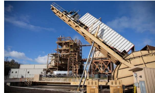
Biomass power Station
